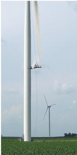
One platform feature includes positive locking to the tower to provide greater stability even at the fullest 20 ft/6.2M extension at maximum rated wind speeds. Taking serviceability into the design plan, Power Climber Wind proactively integrated easily accessible and removable cabling and components for faster platform maintenance, as well as added elements to ease transportability from site to site.
