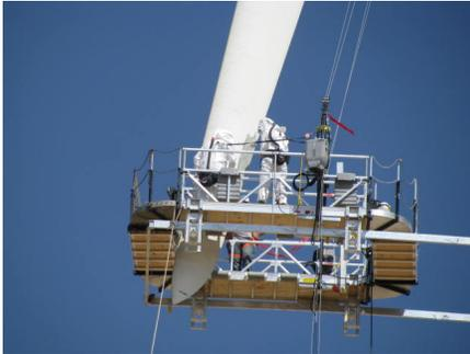
Seattle – Spider, a division of SafeWorks, LLC, has supplied their modular suspended access platforms to the Lankford Painting Company to enable their tower and blade repair and inspection jobs on Siemens 2.3 MW towers at four different sites in Texas.
