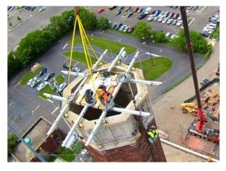
Seattle – Spider, a division of SafeWorks, LLC, recently provided a custom suspended scaffolding solution for tuck-pointing and brick repair work on the 125-ft tall chimney stack at Lane Tech High School in Chicago.
